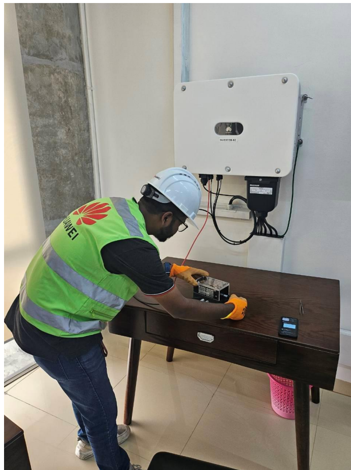
Figure: On-site AFCl testing by Huawei Service Engineer
