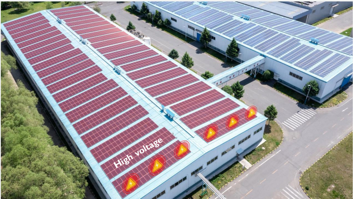
Figure 9. High voltage on the rooftop
