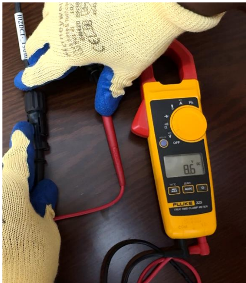
Figure: After remote shutdown the string voltage is 8.6V DC (&gt;30V DC)
