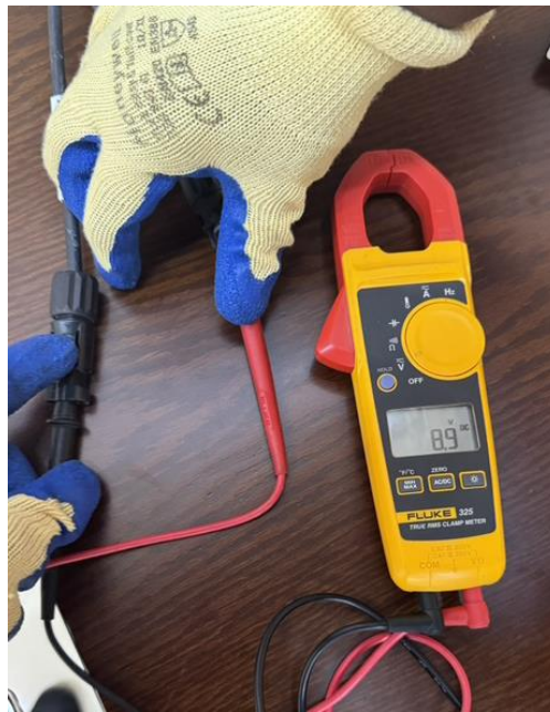
Figure: After DC switch turned off the string voltage is 8.9V DC (>30V DC)
